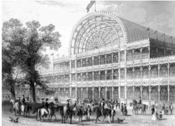
Exhibit I : The façade of the original Crystal Palace, London (1851)
